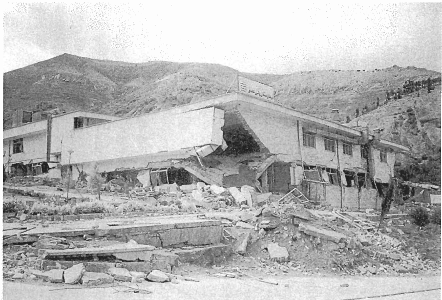
Failure of Vali-asr hospital, Rudbar
